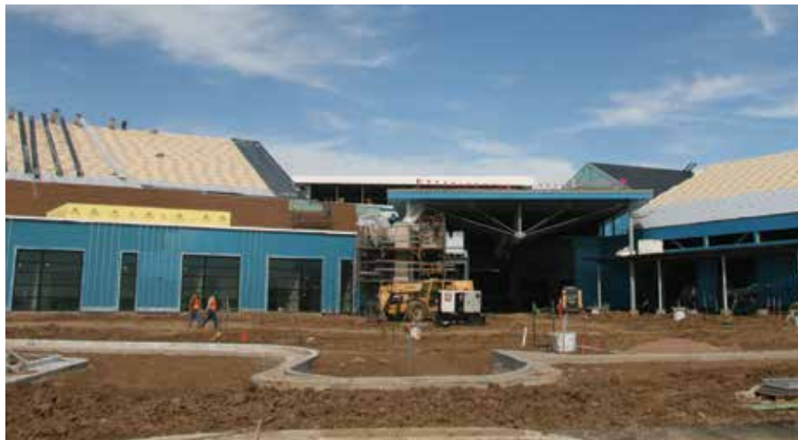
Main entrance work at Bison Ridge
